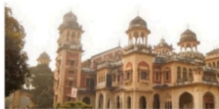
Figure 1. Structural view of Senate hall building, Allahabad University, India.
