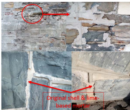
Figure 1. Recent repairs (Robben Island, 2019)
