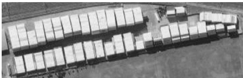
Figure 3. Example of the unique shape and size of shipping containers. Source: Google Maps.
