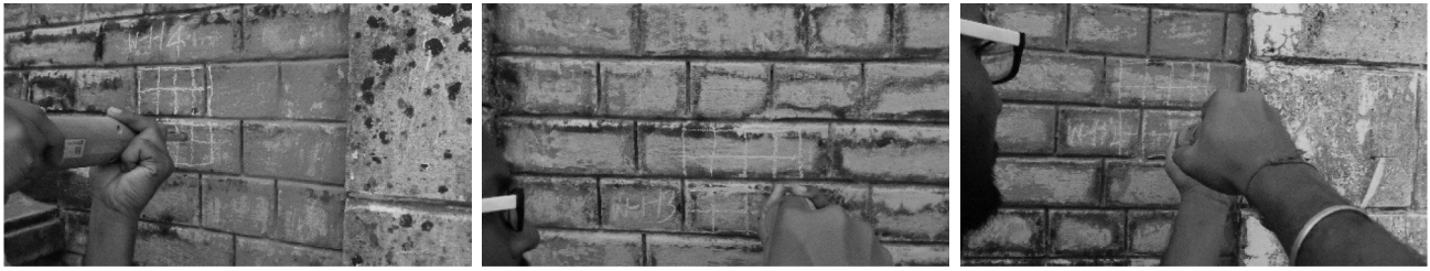
(a) Identified locations of WoP masonry walls
