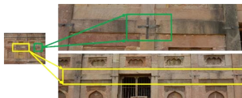
Fig. 7 Connection element used in Mughal tombs
