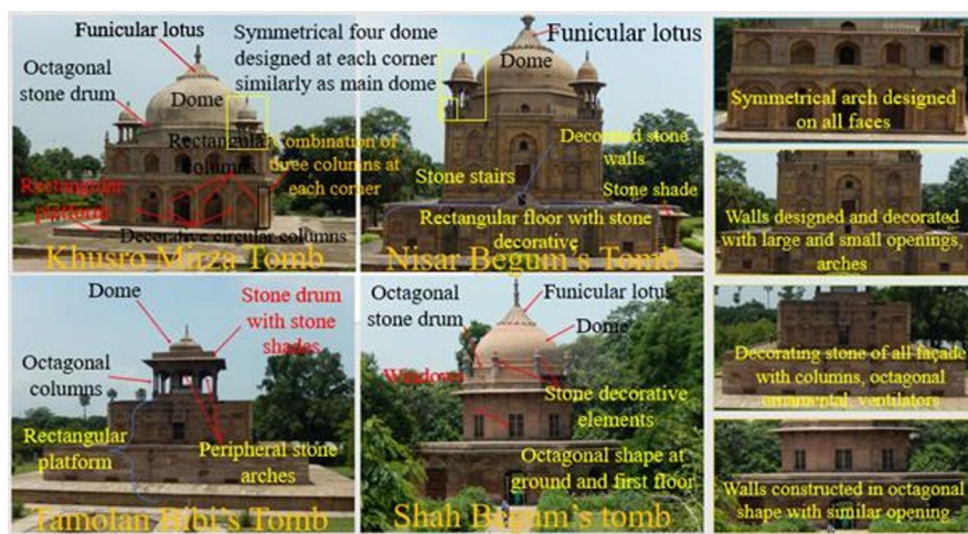
Fig. 2. Structural view of Khusro Bagh tombs
