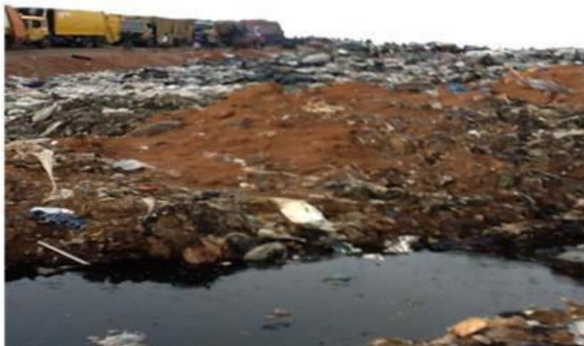
Figure 2. Photograph of part of the Olusosun landfill site showing areas of refuse dump and leachate release.
